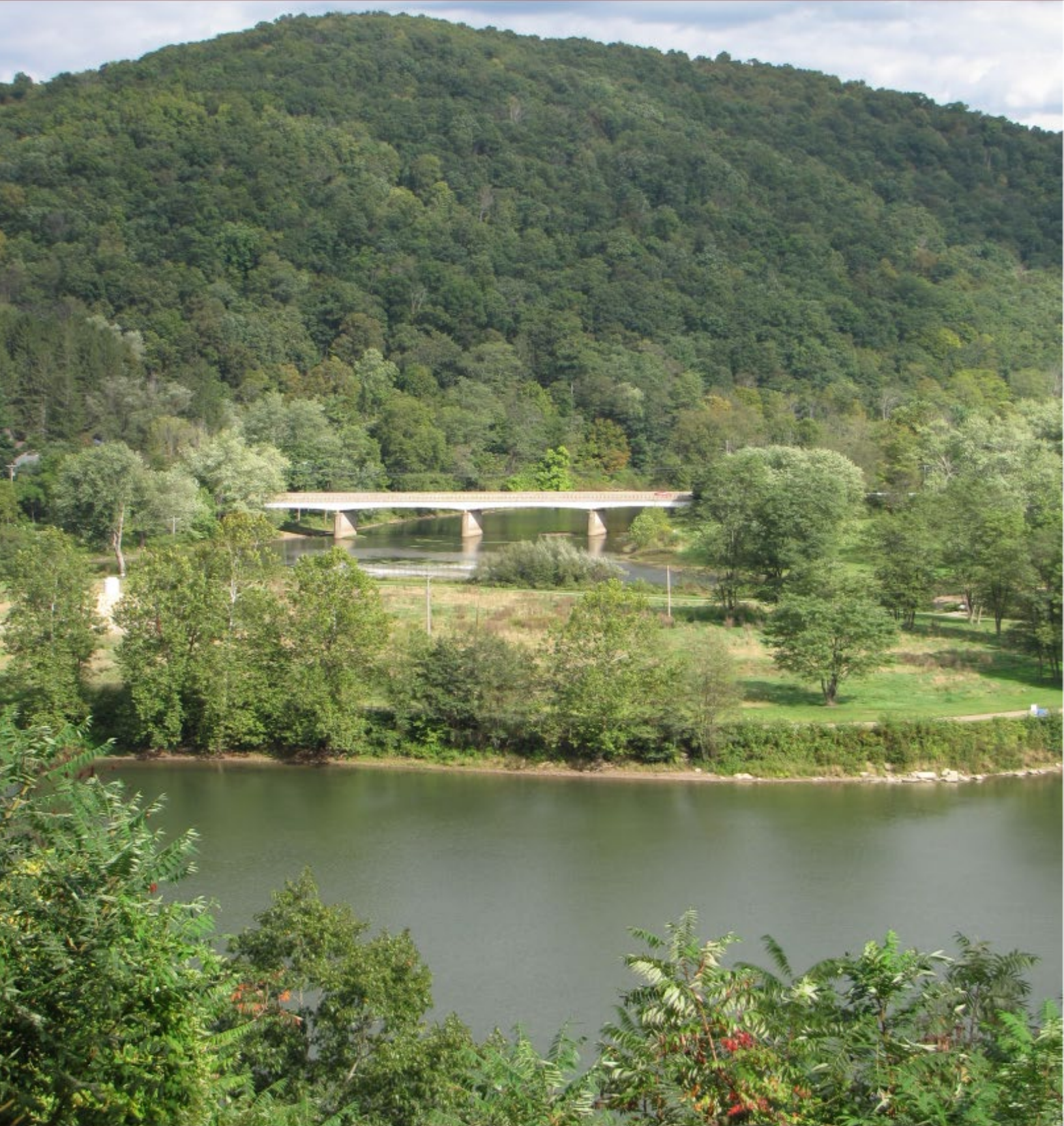
PA 36 over the Allegheny River in Forest County
