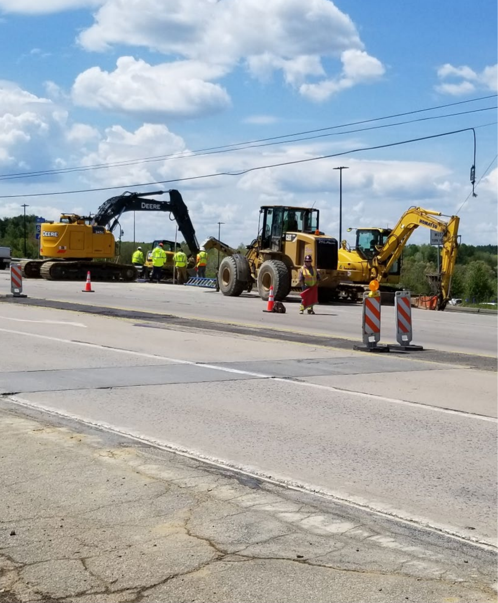
Safety and Intersection Improvements along PA 68 in Clarion County
