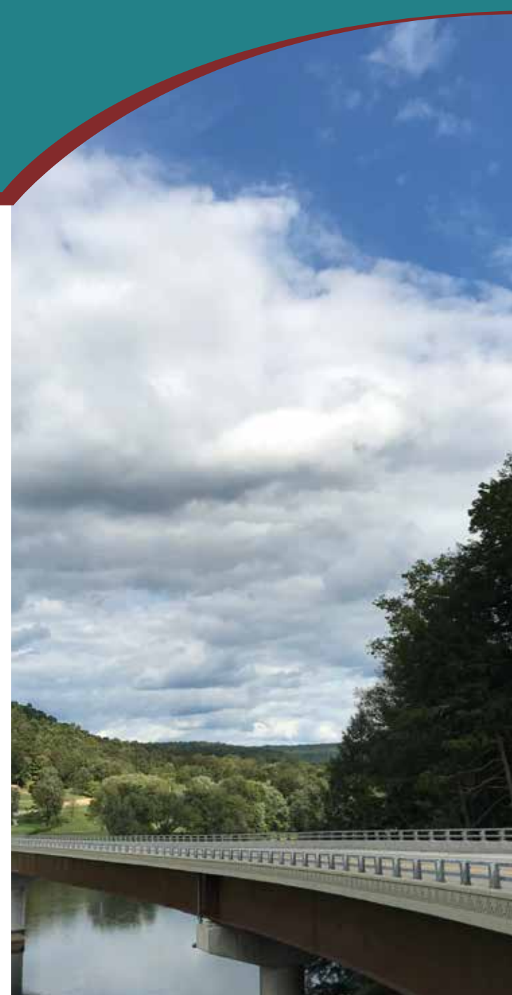
US 62 over the Allegheny River, Tionesta Township, Forest County
